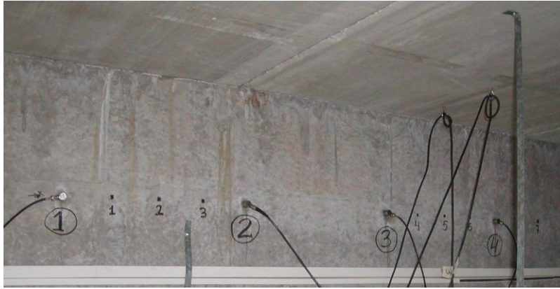
Figure 6. Examination of a reinforced concrete beam.
